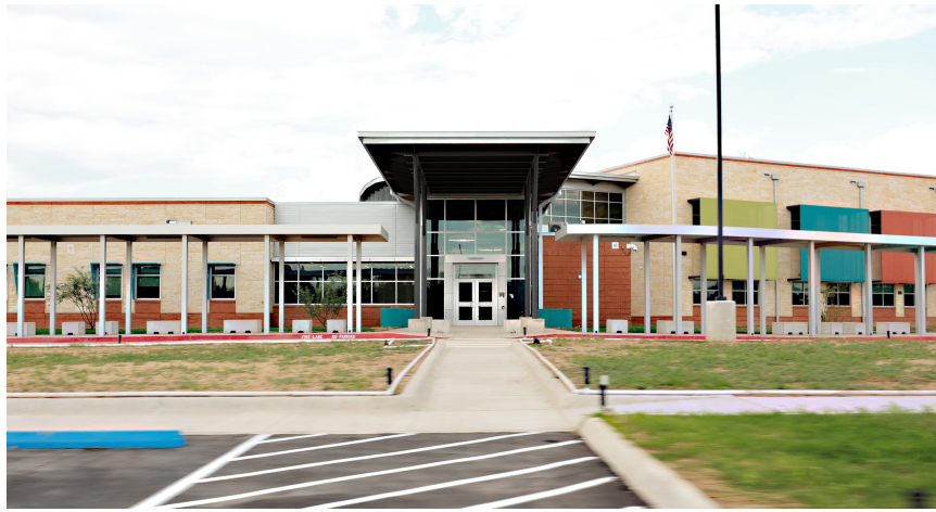
Legacy Elementary School in Uvalde, TX (Prestamos CDFI NMTC 2024)
